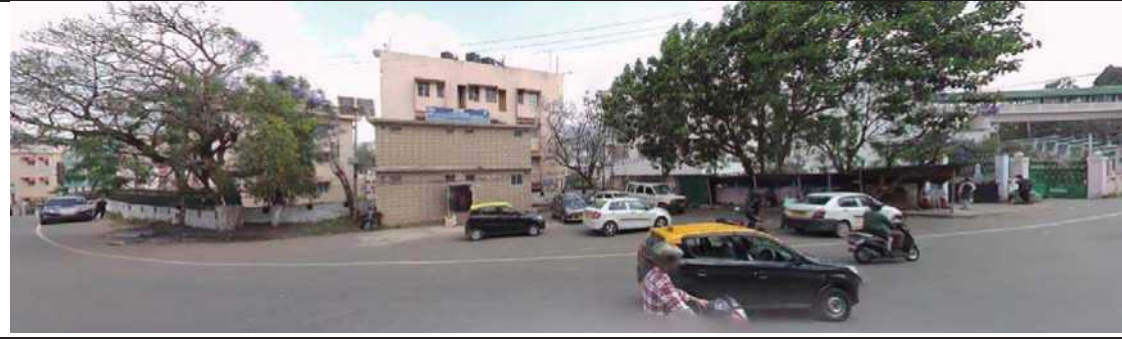
Vivekananda Road – MLCP Site existing situation
