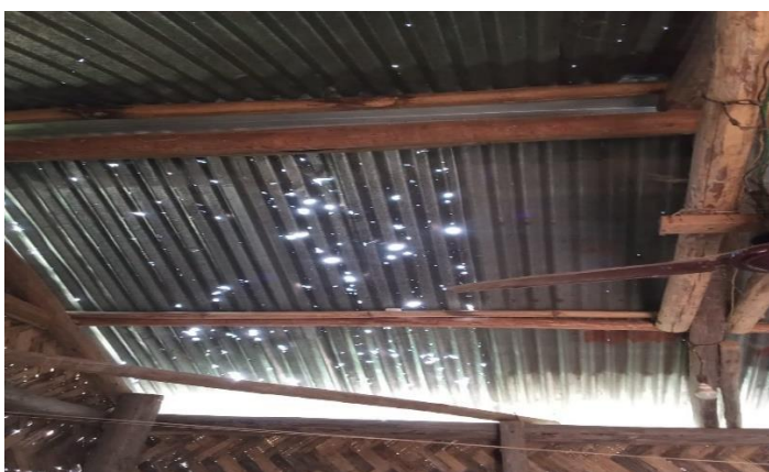
Houses damaged due to Hailstorm at Rongchekgre & Nengkong villages under Bahgmara C&RD Block, South Garo Hills District
