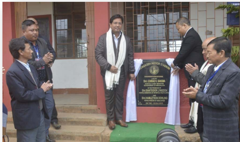
The Chief Minister also laid the foundation stone for the construction of the Nongkseh Indoor Stadium in the presence of local M.L.A. and Minister Urban Affairs Hamletson Dohling on the 20th of December 2019.
